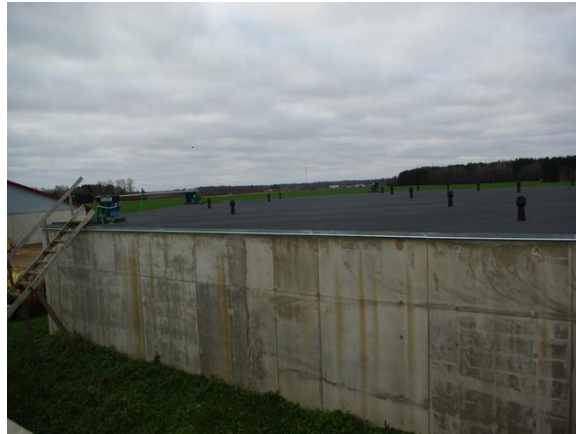
Joonis 4. Jäiga kattega rõngasmahuti (foto A. Nõmmeots) Figure 4. Ring shaped manure storage with permanent high wall (to 4 m) (photo A. Nõmmeots)
